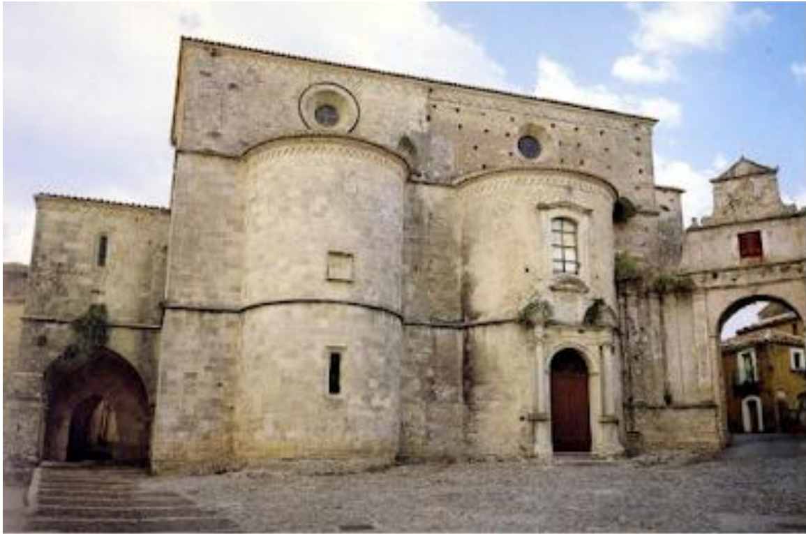
Gerace (Ierax). The former Orthodox cathedral in Gerace, Calabria
